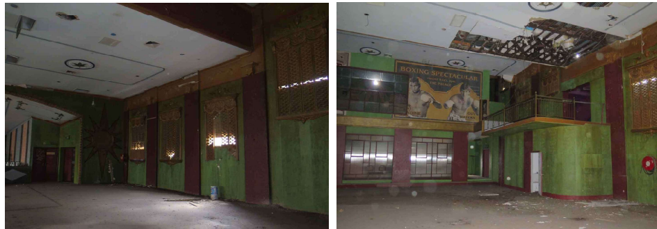
Figure 23 – Homebush Theatre, First Floor Interior, looking to the eastern wall with grilles over the windows (left). View looking south towards the entry vestibule. The original ceiling finish has been removed and covered in plasterboard (Source: NBRSArchitecture, October 2016)
