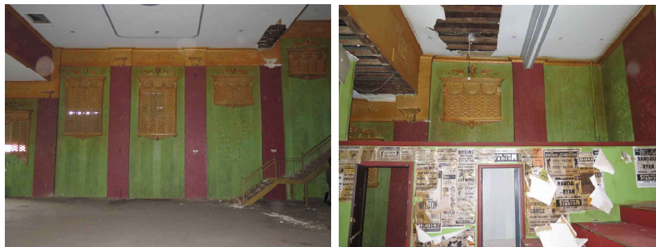
Figure 26 – Homebush Theatre, First Floor Interior, showing the later addition concrete slab flooring and stair and balustrading leading to the bar area above. The height of windows indicates the original raking of the flooring. At right, upstairs bar area (Source: NBRSArchitecture, October 2016)
