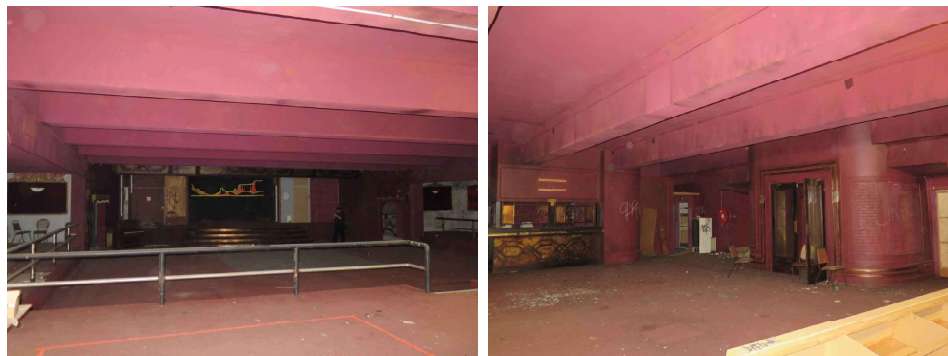
Figure 19 – Homebush Theatre, Ground Floor, showing the later addition reinforced concrete slab with exposed beams that date to the removal of the original raked floor that formed part of the original theatre configuration. View north, at left, shows a "mosh pit" and modified stage with the concrete slab horizontally dividing the proscenium. At left shows the entry and foyer (Source: NBRSArchitecture, October 2016)
