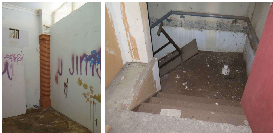
Figure 24 – Homebush Theatre, Ground Floor Entry, showing an extant candy-twist column, possibly dating to the 1930s, partially concealed by later additions to the theatre. The fire stair (at right) shows evidence of an altered layout (Source: NBRSArchitecture, October 2016)
