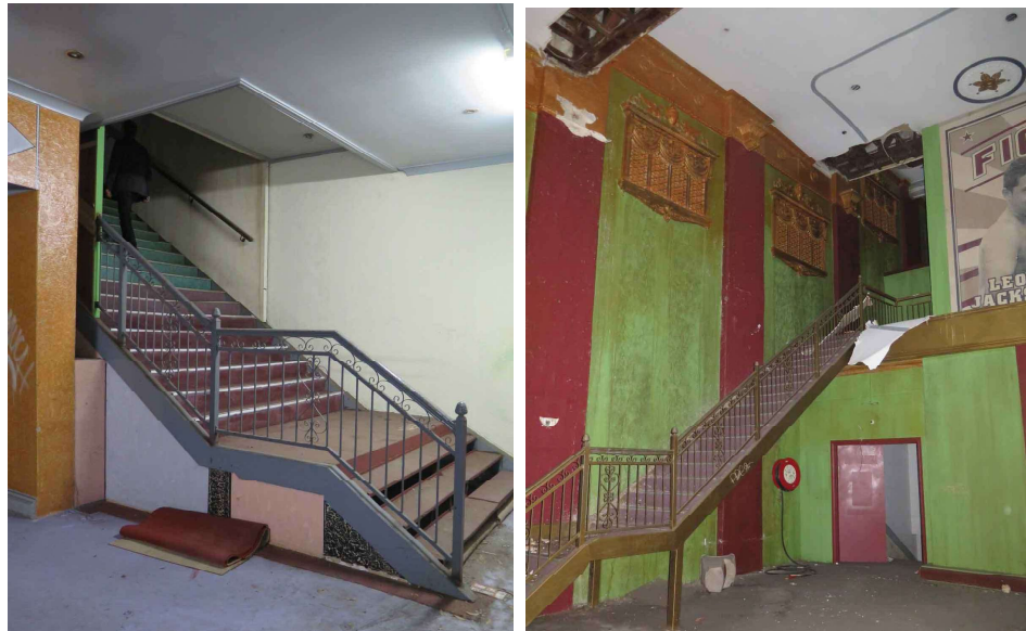
Figure 25 – Homebush Theatre, First Floor Interior, showing the later addition concrete slab flooring and stair with balustrading leading to the bar area above. The height of windows indicates the original raking of the flooring (Source: NBRSArchitecture, October 2016)
